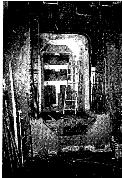
Figure 3. Self compacting concrete
