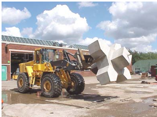
Figure 12: Handling of Xbloc ® armour unit
