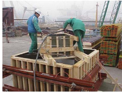
Figure 5: Vibrating of concrete in the mould
