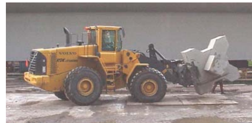
Figure 11: Handling of Xbloc ® armour unit
