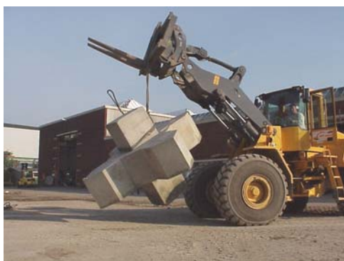
Figure 13: Lifting the Xbloc ® with a sling.
