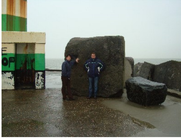
Figure 2. 45 tons cube and toe rock displaced from breakwater front (IJmuiden, The Netherlands).
