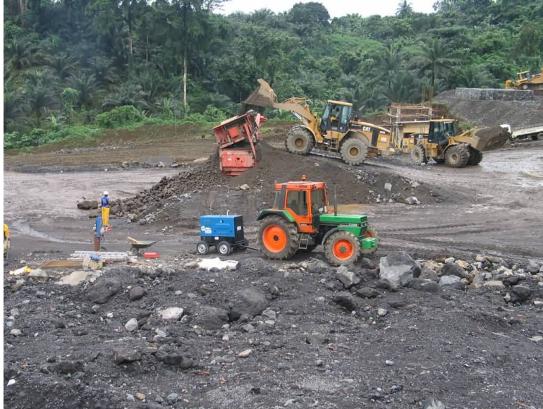
Figure 1. Separating fines from core through a grizzly at Limbe, Cameroon.
