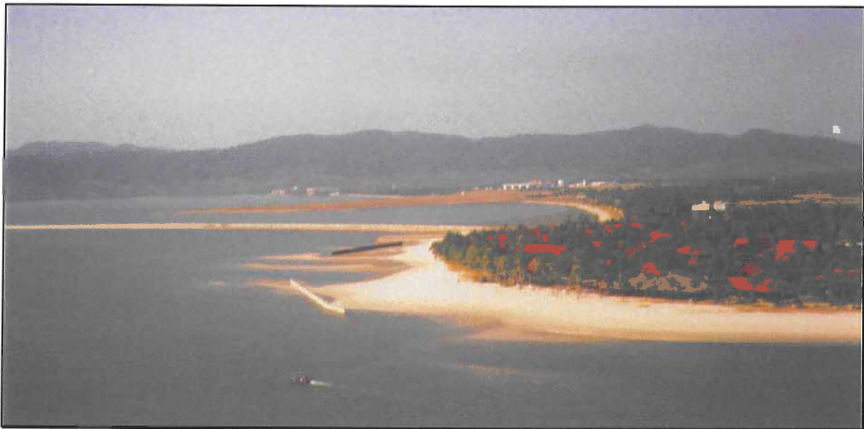
Photograph 4. Overview of the beach resort with pile rows.
