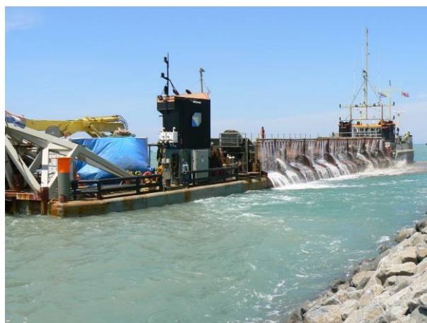
Figure 15: Rock dumping with Arca
