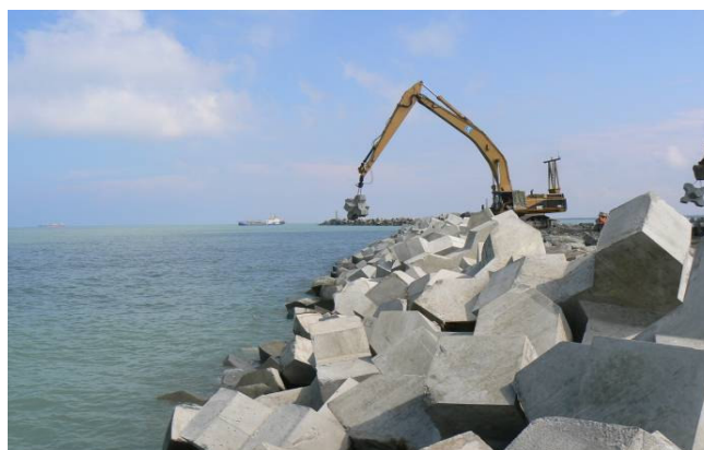
Figure 16: Xbloc placement
