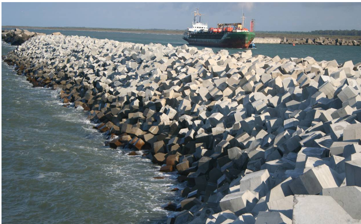
Figure 17: Impression of completed rehabilitation works
