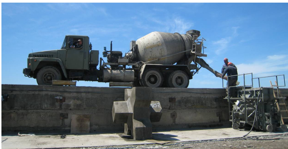
Figure 11: Pouring Xbloc from concrete mixing truck
