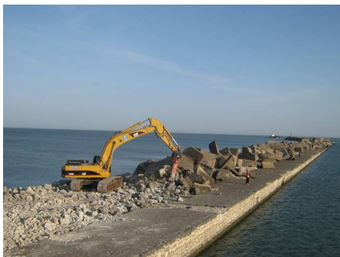
Figure 14: Impression of Rock Hammering
