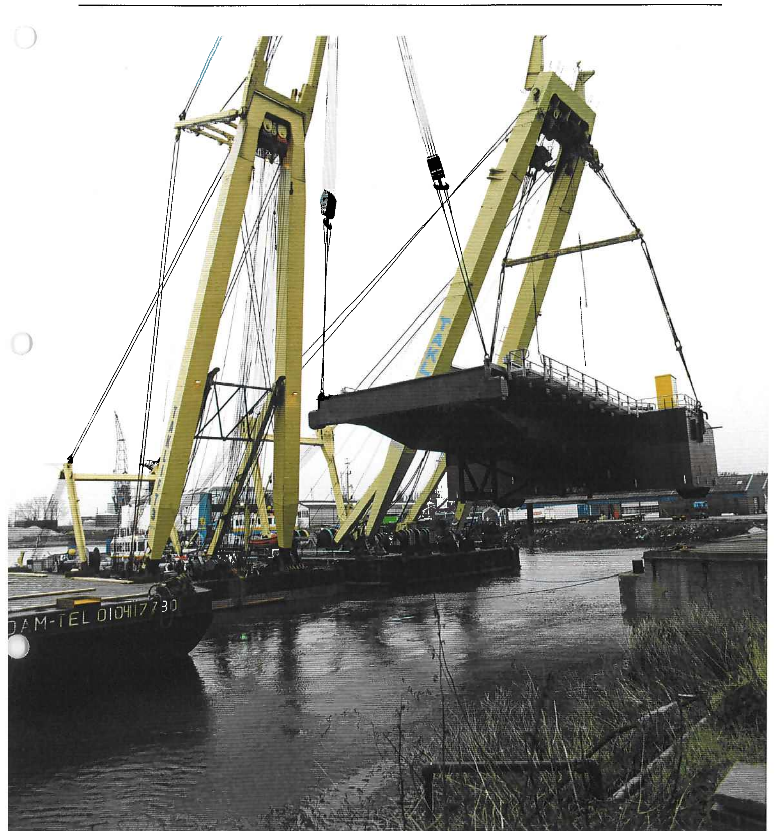
fig. 13 Loadout of the Ro-Ro pontoon
