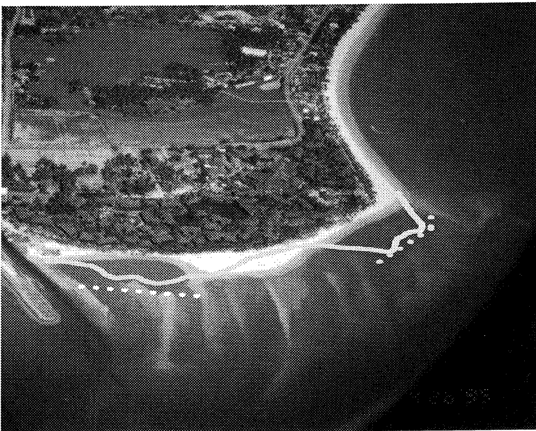
Photograph 6. Situation before and after construction of pile rows
