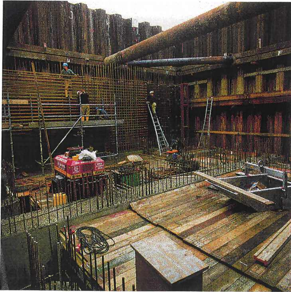
Figure 10 Construction works pump station
