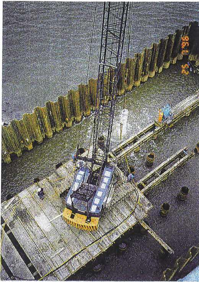
Figure 8 Pile driving from temporary bridge
