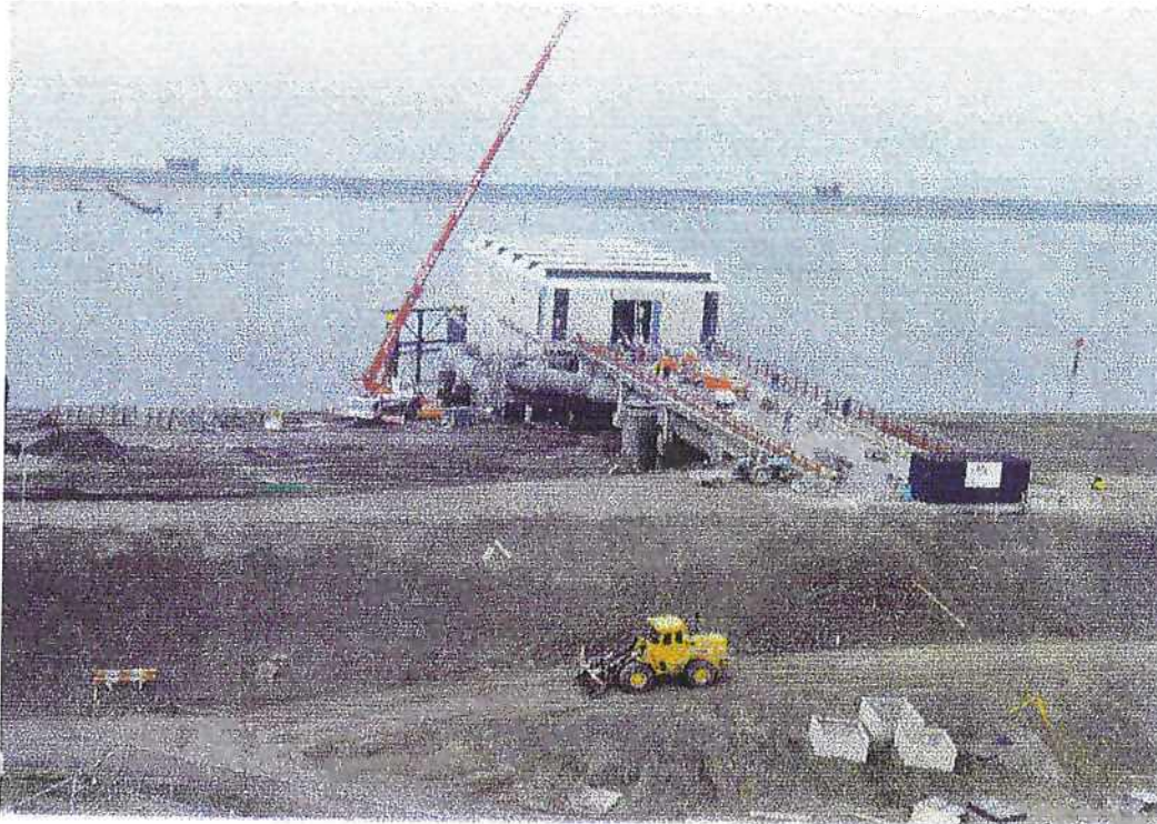
Figure 4 Overview construction activities
