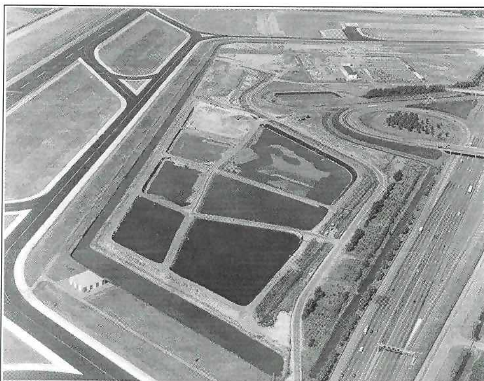
"Water Storage at the airport area"
