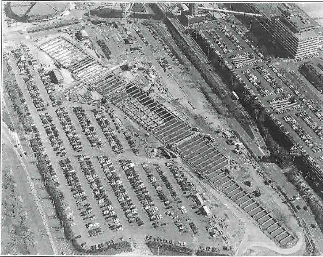
"One of the pits near the connection part"
