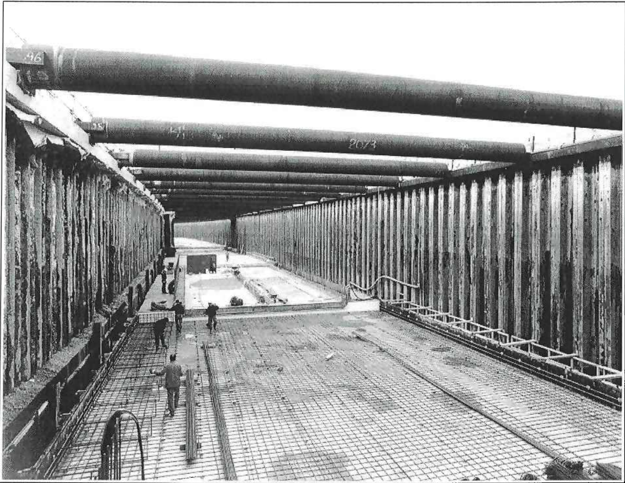
“View inside the dock after transport of the immersed elements”
