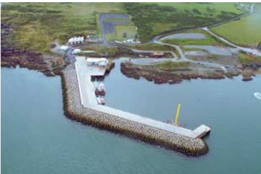
Fig. 9 First completed Xbloc breakwater in Europe: Port Oriel Ireland.
