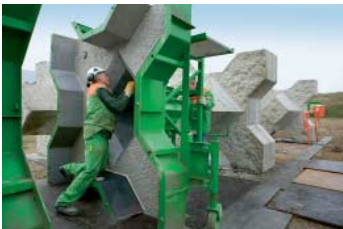
Fig. 5 The Eco Xbloc mold and a freshly cast Eco Xbloc.
