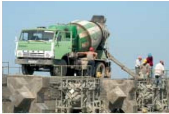
Fig. 7 Filling of molds directly from the truck mixer.
