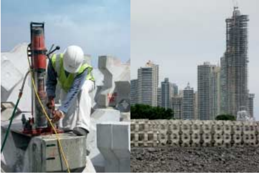
Fig. 8 Extracting cores at Cinta Costera Panama and storage area.
